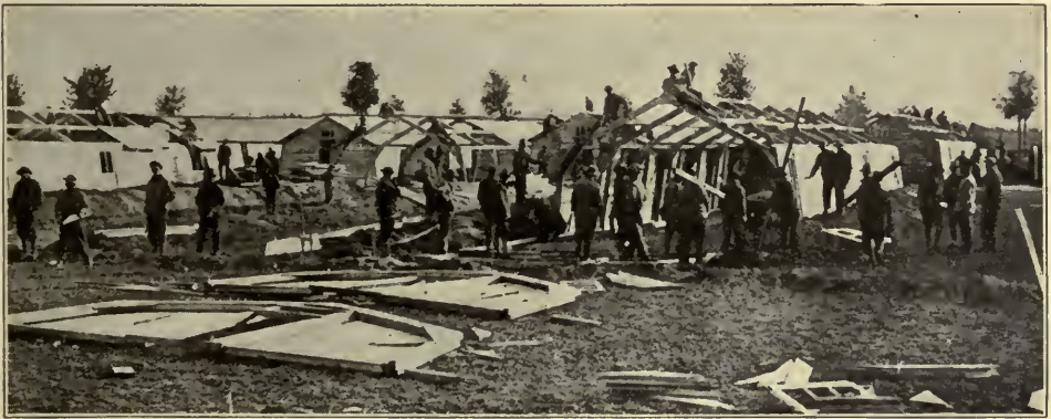
ENGINEERS ERECTING A CANTONMENT IN FRANCE
