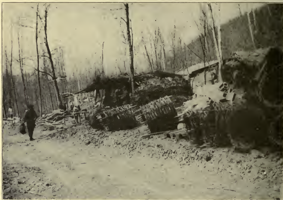
A FIELD FORTIFICATION SUPPLY POST
